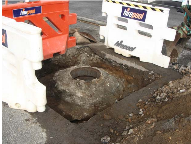
Photograph 9: Top off manhole, and preparing to install fiberglass liner.
