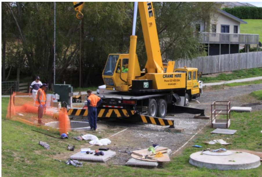
Photograph 9: Top off manhole, and preparing to install fiberglass liner.
