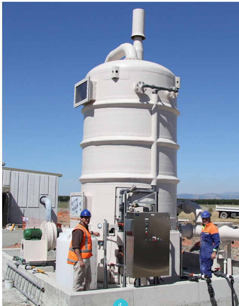
4: Armatec Biological Scrubber in Pines II WWTP, Christchurch removing >99% of 11-42 ppm H 2 S 5: Inorganic packing media used for microorganisms
