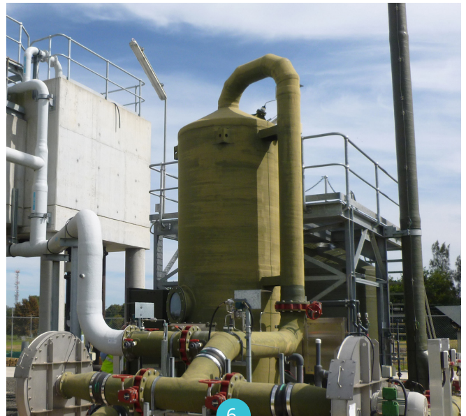
6: Armatec-designed Biological Scrubber at Richmond WWTP. 7 & 8: Armatec BSCB Plug & Play unit installed in Motueka WWTP, New Zealand removing >99% of 20-100ppm H 2 S at 0.2m 3 /s.
