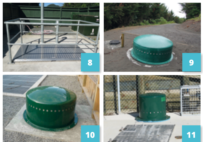
8: Sealing pump station lids are needed to guarantee no odours. 9: Large Green Dome® GDOF-72 for air released from long rising main. 10: Larger Green Dome® positioned away from pump station out of way of service crews. 11: Smaller Green Dome® positioned on top of pump station.
