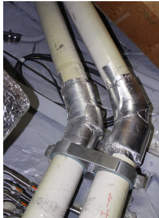
WhispaPipe with butt and strap joints, and acoustic insulation reinstated with aluminium tape.
