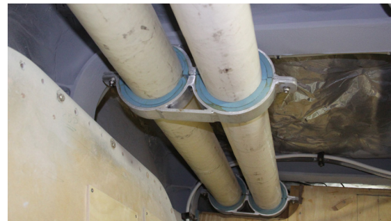
WhispaPipe, with factory fitted acoustic insulation minimises on-vessel installation time and costs.
