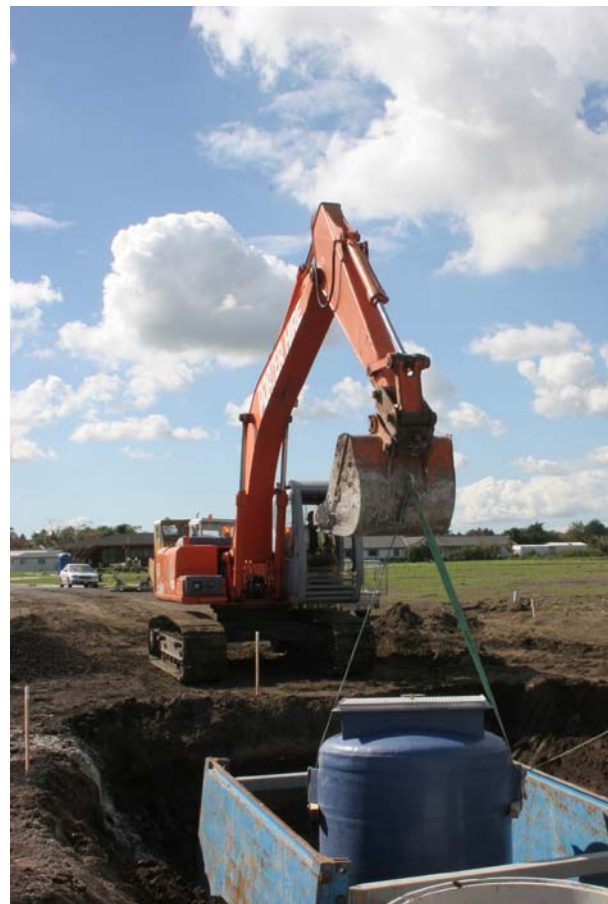
All fibreglass pump station fitted with a FLYGT TOPS Base being lowered into position in municipal subdivision. Hole dug, pump station installed and backfilled in just one day. DVD available on request.
