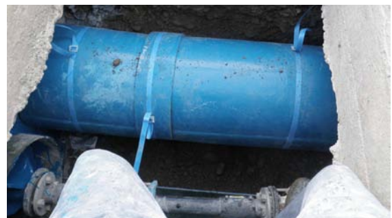
First 'Carrier Pipe' installed.
