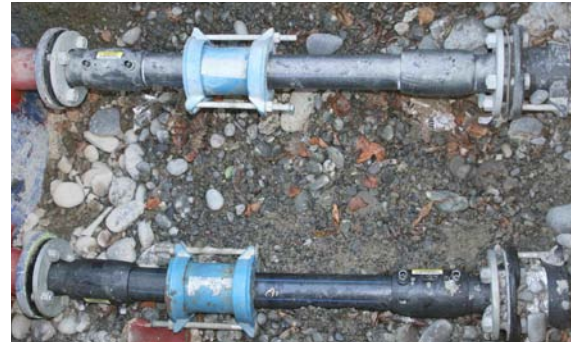
HDPE pipe before 'Carrier Pipes' installed.
