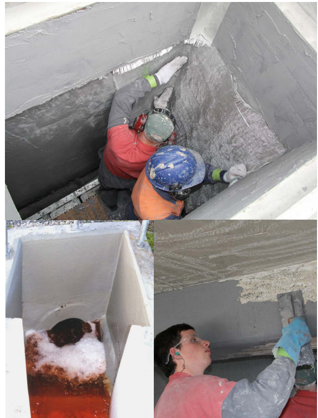
Armaline® coatings are used to protect concrete surfaces from hydrogen sulphide attack in wastewater applications such as pump stations and inlet works.
