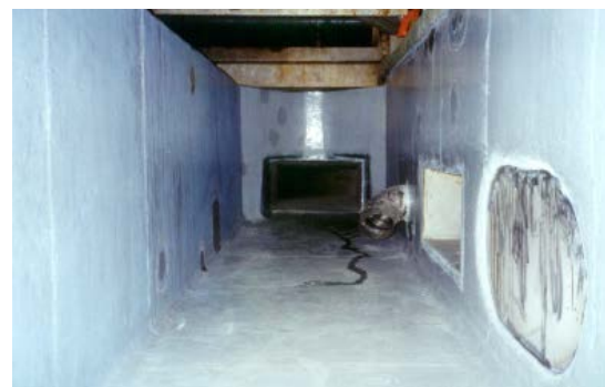
Armaline® Chestline under paper machine applied in tight shutdown period; concrete was not able to be 100% dried.
