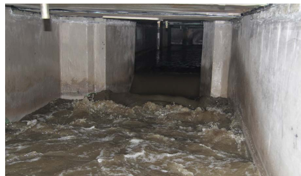
Armaline® Chestline under paper machine applied in tight shutdown period; concrete was not able to be 100% dried.
