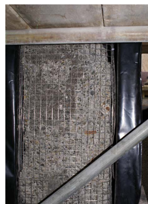
ArmaGrout used to rehabilitate concrete before protective coating applied. Replacement steel reinforcing was added to structural concrete column (left) before ArmaGrout pour. Leaking concrete chemical bund wall (right) sealed and restrengthened using ArmaGrout.
