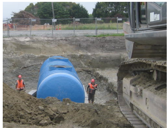
Light weight horizontal surge tank is easy to transport and install.
