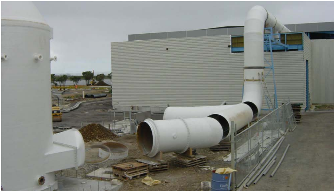
Ventilation system at biosolids plant at wastewater treatment plant during installation. Duct support structures are pre-installed for elevated ducts, but at ground level temporary supports can be used first, and permanent supports installed later.
