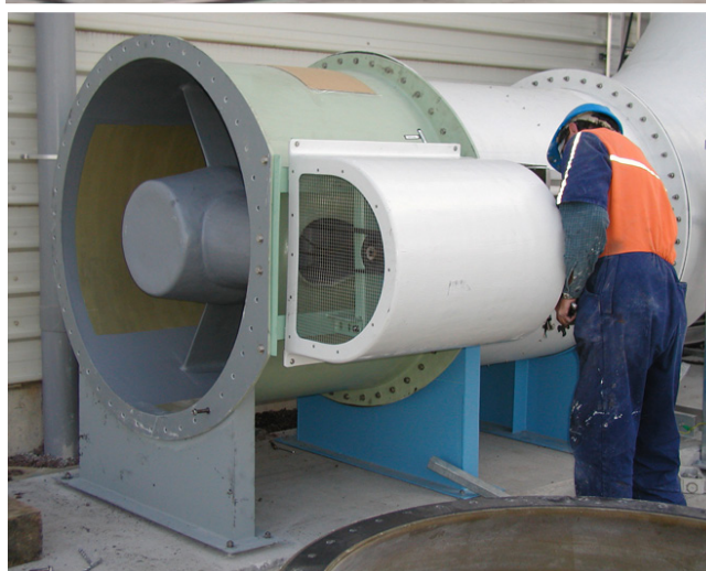
Left: Axial fans, duty and standby, providing fresh air to biosolids processing building at WWTP. Right: Large and small centrifugal fans being assembled ready for despatch.
