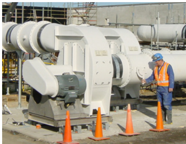
Fibreglass fans handling air with hydrogen sulphide at wastewater treatment plant on the coast.
