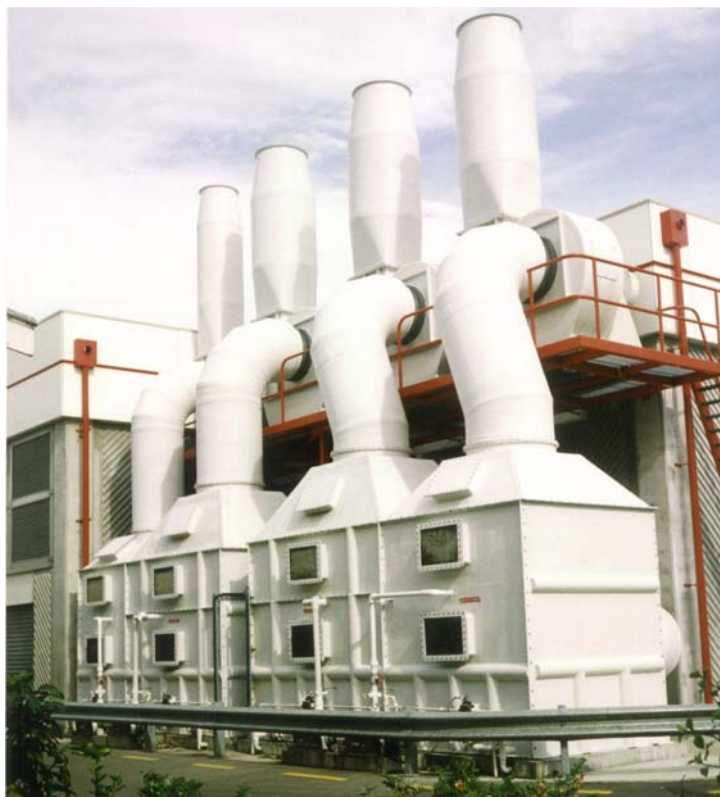
Top left: Two stage horizontal packed bed scrubber for tannery odours.
