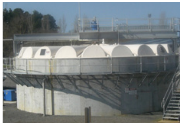
Segmented barrel vault cover over fermenter tank, Ballarat, Australia.
