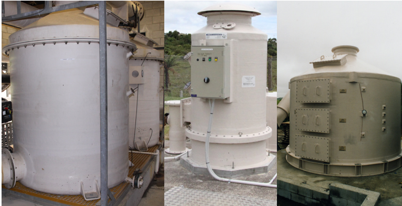
Carbon bed adsorbers for H_2S and other volatile organic gases, all force ventilated with fans.
