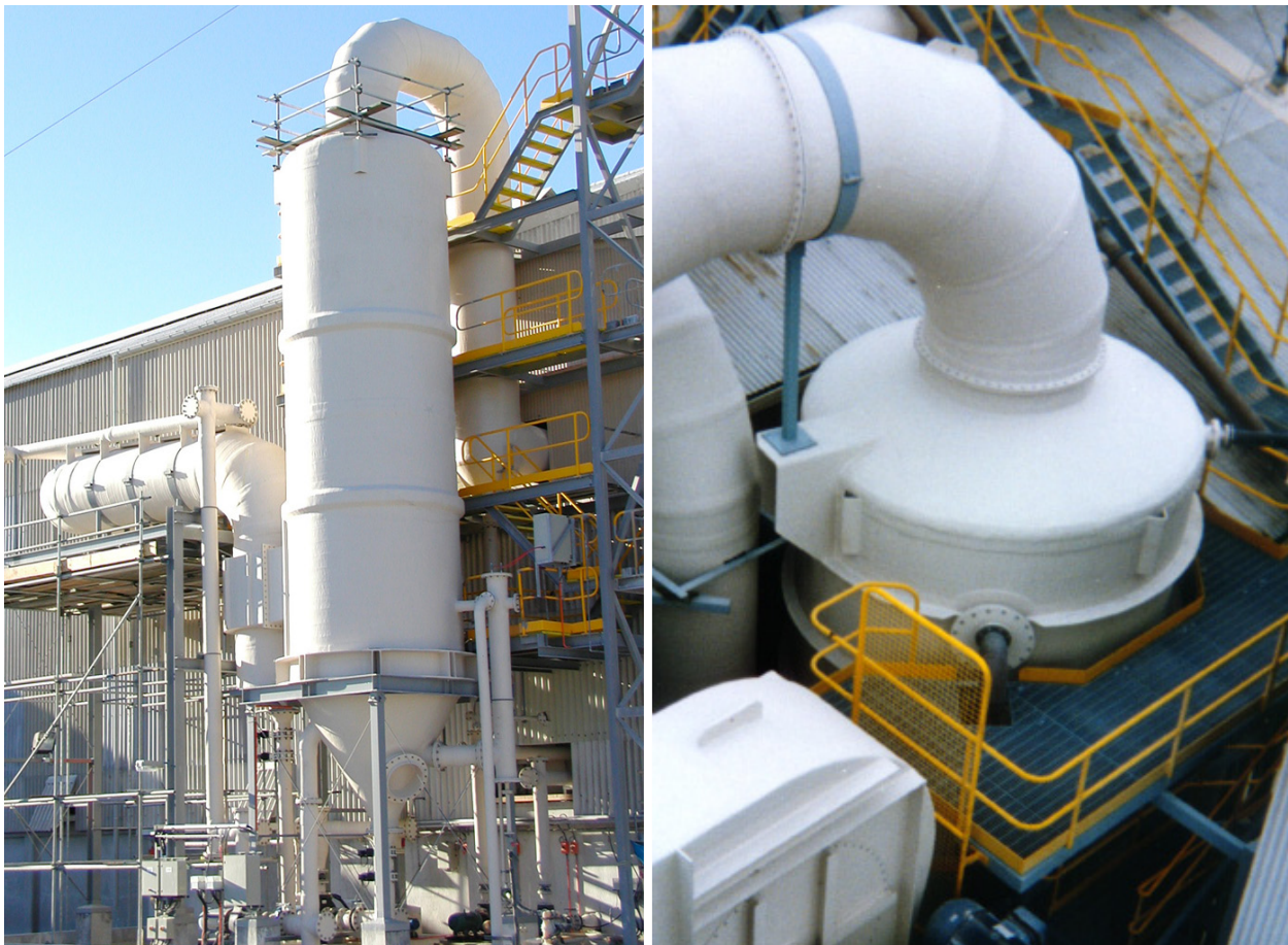
Void tower scrubbers at fertiliser plants, for removing fluoride gases. Silica deposition requires use of void tower scrubbers.
