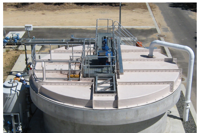
Flat segmented cover over clarifier tank, Sunset Coast, Australia.
