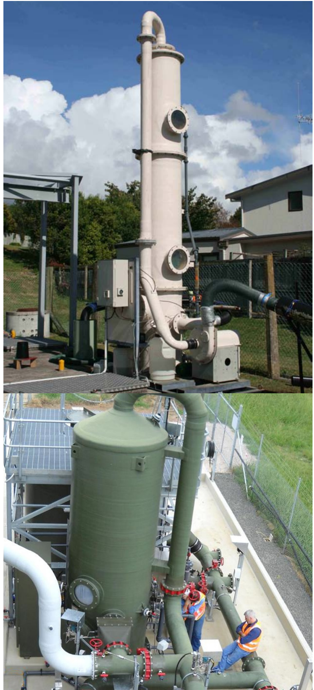
Left: Biological scrubber removing H_2S . Top right: Biological scrubber pilot plant at pump station. Bottom right: ARMATEC designed biological scrubber at Sydney WWTP.
