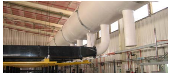
Plenum style header and branches
