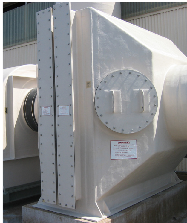
Left: Wet cyclone at fertiliser plant, for removing liquid droplets after void tower scrubbers. Right: Kimre mist eliminator removing acid droplets and water mist from air stream.
