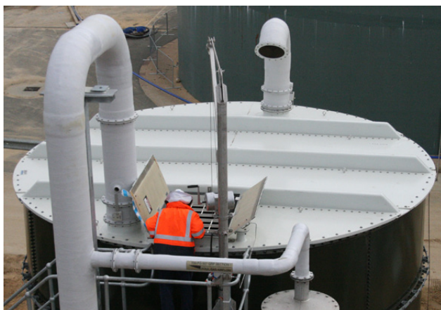
Top left and right: Removeable segmented covers over inlet chambers and PST tanks at wastewater treatment plant. Bottom left: Removeable cover over tank at wastewater treatment plant. Bottom right: Covers over pulp washers at pulp and paper mill.
