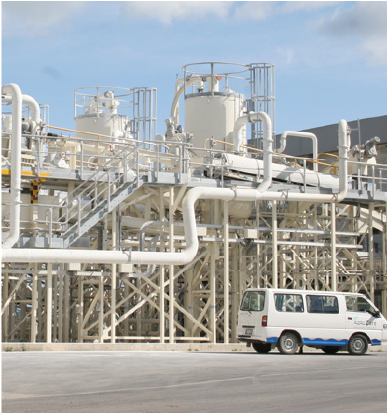
Ventilation system at biosolids plant at wastewater treatment plant. Fibreglass ducts connect to strategic process points to collect dust and fumes. Ducts are irrigated and sloped to flush solids away.
