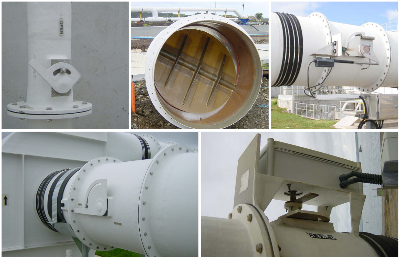
Manual and actuated fibreglass dampers with quadrant handle.
