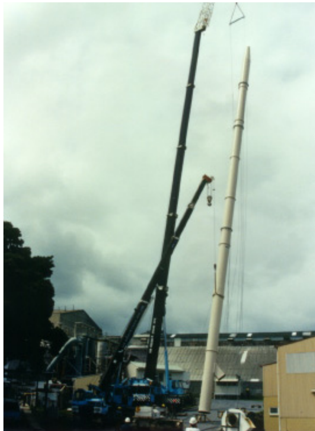
Left top: Fanstack for forced draft cooling tower. Left bottom: Stack for fertiliser plant being lifted into position. Right top: Stack for chlorine fumes at pulp and paper plant. Right Bottom: Stack at WWTP with diffuser.
