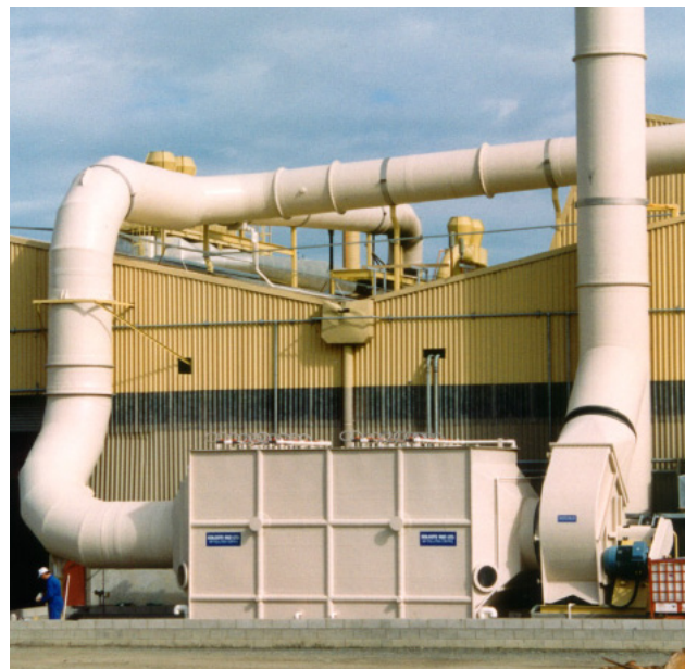
Two-bed horizontal packed bed scrubber removing formaldehyde from press gasses at particle board plant.
