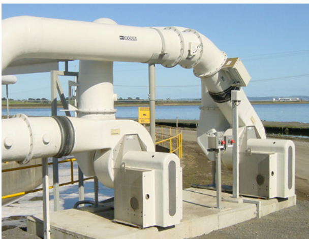
Fibreglass fans handling air with hydrogen sulphide at wastewater treatment plant on the coast.
