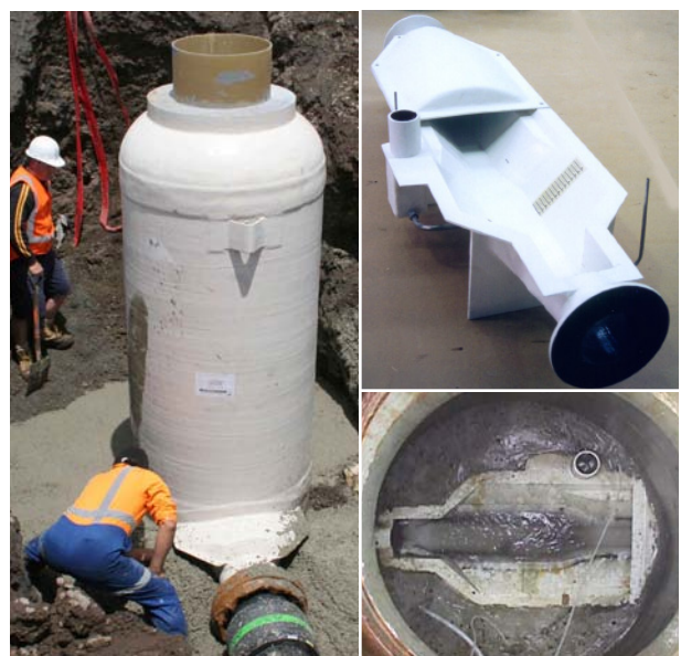
Trapezoidal flumes for flow monitoring in small sewers. Easy to set up with flow sampling.
