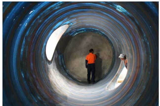
Horizontal surge tank under construction. Pump out chamber is fitted to one end of surge tank.
