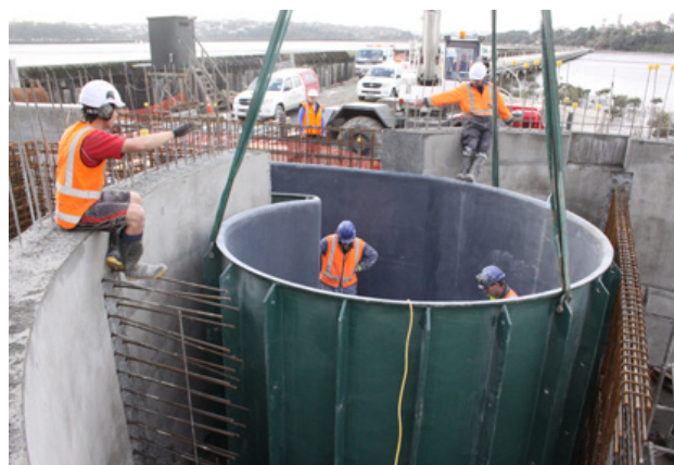
Vortex former lifted into place
