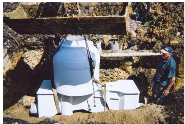
Parshall Flume installed in nine hour shutdown
