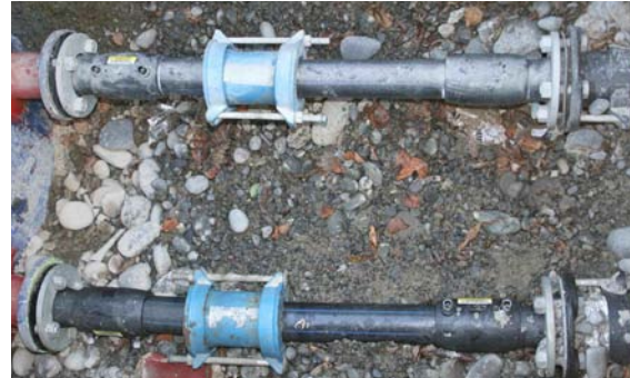
HDPE pipe before 'Carrier Pipes' installed.
