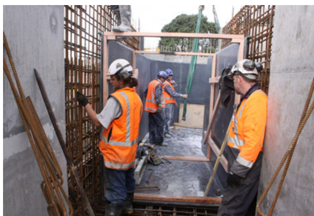
Setting up for concrete to tie to vortex former
