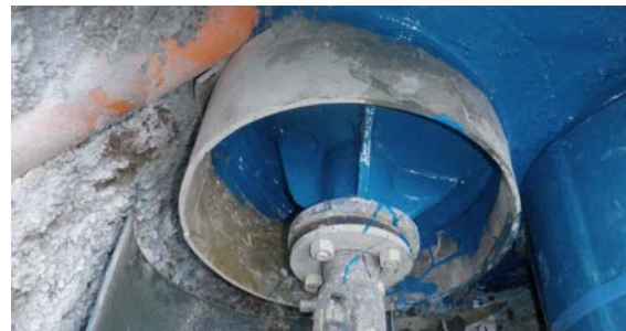
'Carrier Pipe Starter' fitted to pump station end.
