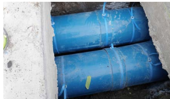
Both 'Carrier Pipes' installed. HDPE pipe is now protected. It has room to move reducing chances of fracture due to ground movement.
