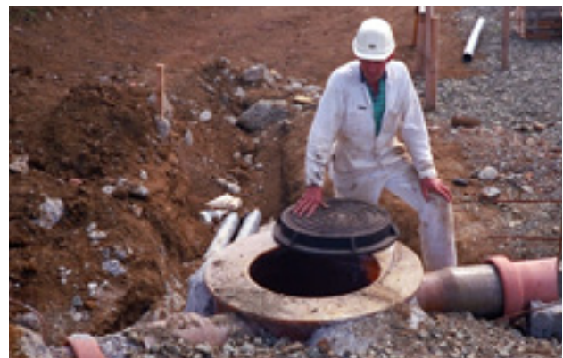
ARMATEC's first dairy industry fibreglass manhole was installed in 1988, and is still in service today.
