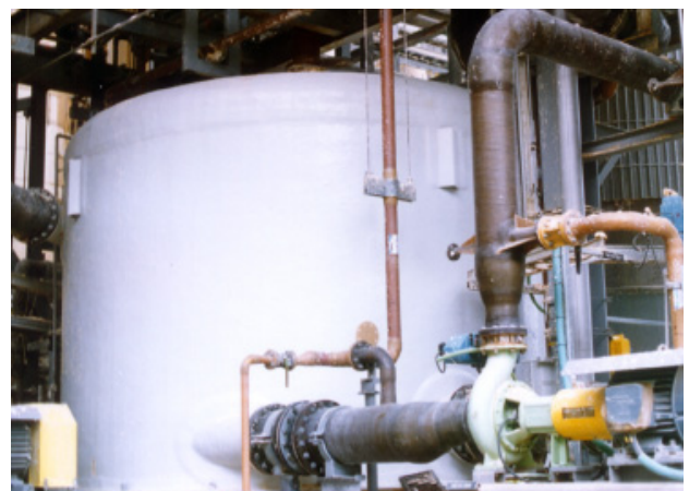
Fibreglass tank at pulp and paper mill, receiving filtrate from paper making process.
