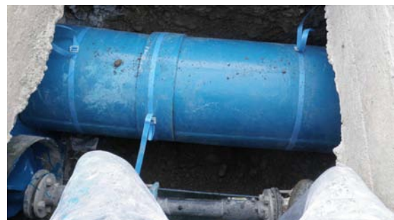
First 'Carrier Pipe' installed.
