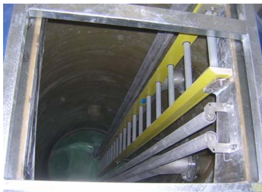
Nozzles, ladders, pump guide rails and discharge pipes are all factory fitted.
