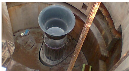
Drop pipe installed before vortex former fitted.
